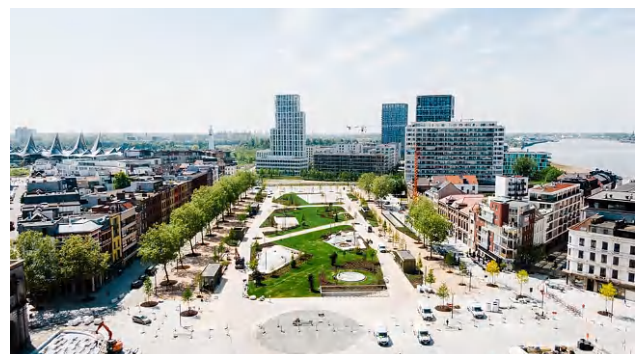
Figure 1: Antwerp Zuiderdokken - cars underground
