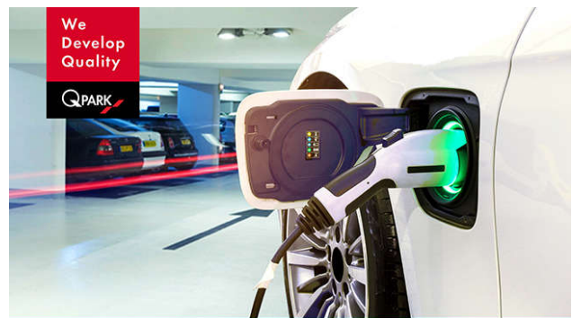
Figure 11: EV charging points
